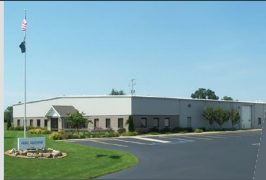
ELCo Enterprises headquarters in Jackson, Michigan
